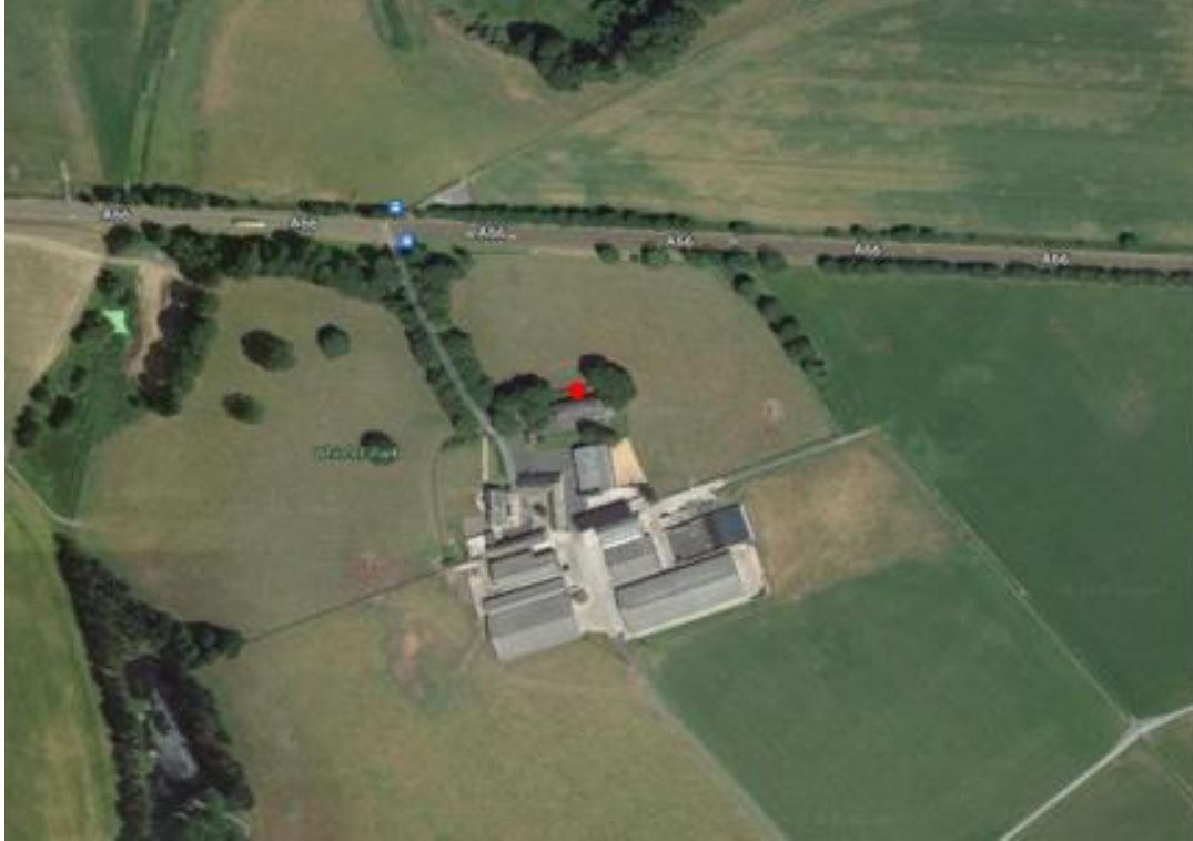
Plate 9: Location of monitoring equipment at Whinfell Cottages
